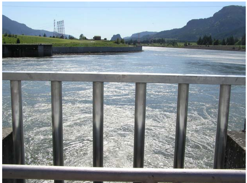
Figure 3b. The large excluder gate is placed in the downstream gate slot with individual partitions
