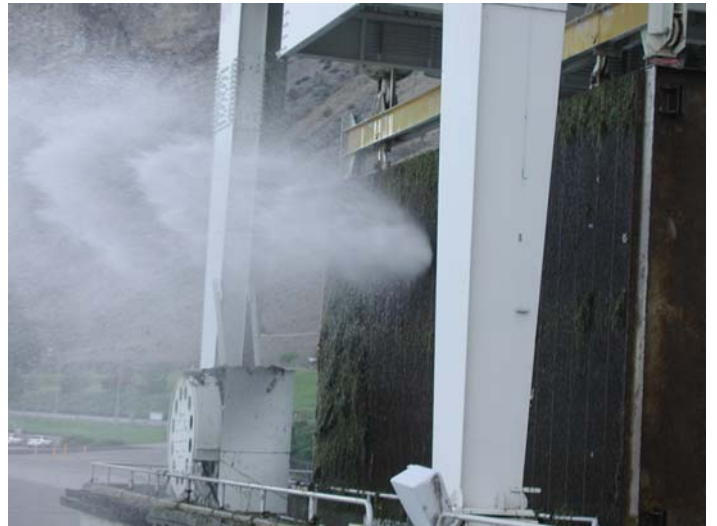
Figure 11d. Large mats of grasses are hosed from the screens during late summer cleaning of the intake valves a Rocky Reach Dam.
