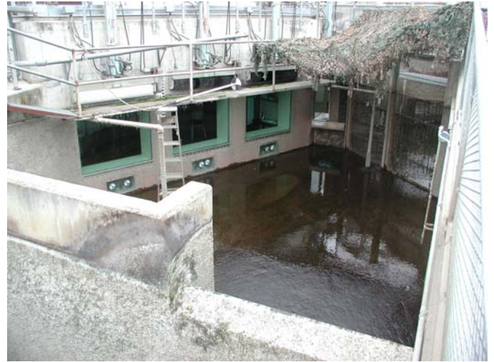
Figure 6b. The adult fish counting station is located upstream from Figure 6a. Note the camouflage netting which is used to cut down the direct sunlight into the fish counting slot.
