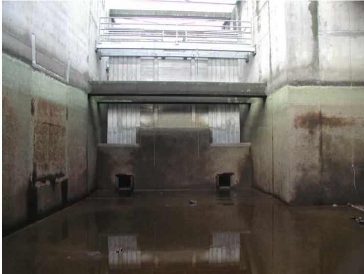
Figure 7a. These photographs show the extended weir crests at the 1 st fish ladder weir located above the Junction Pool at the South shore of the Project. This whole area will be modified prior to the 2006 adult fish passage season.
