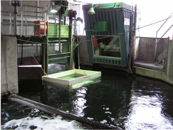
Figure 8a. Old Right Bank fish counting station and last fish counting board on the Columbia River; removed from this Location in mid July 2005.
