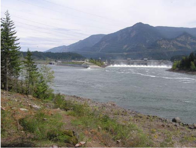
Figure 1a. Bonneville Dam looking upstream into junction to spillway and into junction leading to the New Powerhouse.
