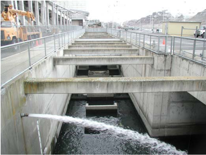
Figure 6a. The 1 st fish ladder weirs above the junction pool may be modified similar to the Lower Granite planned modifications that will be installed this winter, 2006. This modification should reduce fallout rates from the fishway, and, and in the long run reduce time to pass a facility and reduce mortality.
