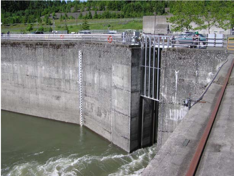
Figure 3a. Sea lion excluders are placed in the new powerhouse entrance gates in mid to late May to keep these mammals outside the actual fishways.
