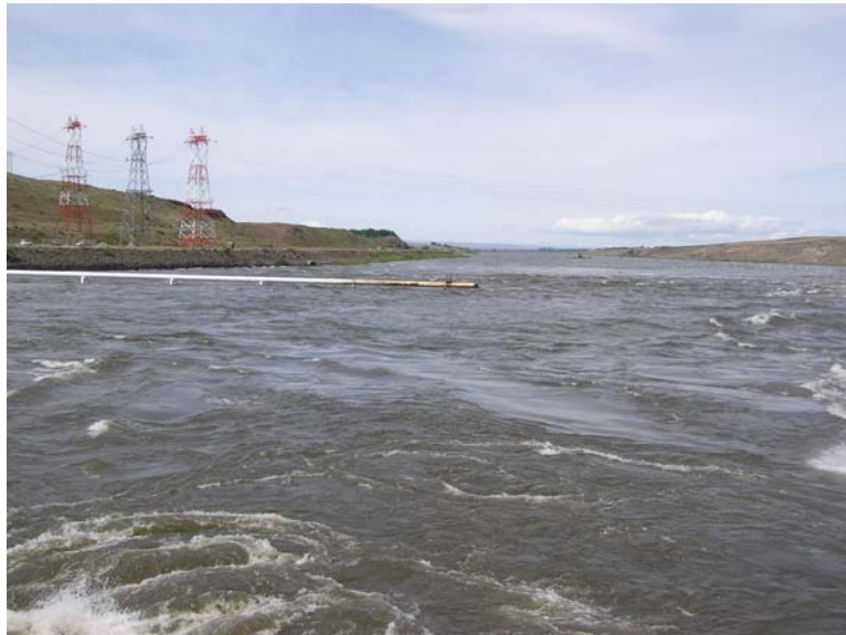
Figure 5c. Note the location of the juvenile bypass outfall pipe looking downstream from the powerhouse deck (unit 6) at Ice Harbor Dam. Photo taken May 05.
