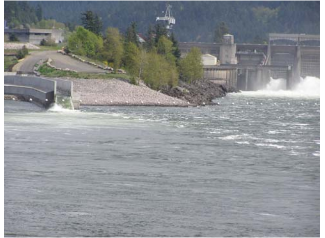
Figure 1b. Bonneville Dam looking upstream to new juvenile bypass outfall from the Corner Collector at New powerhouse and upstream to the the Cascades Island adult fishway entrance located at the north end of the spillbasin.
