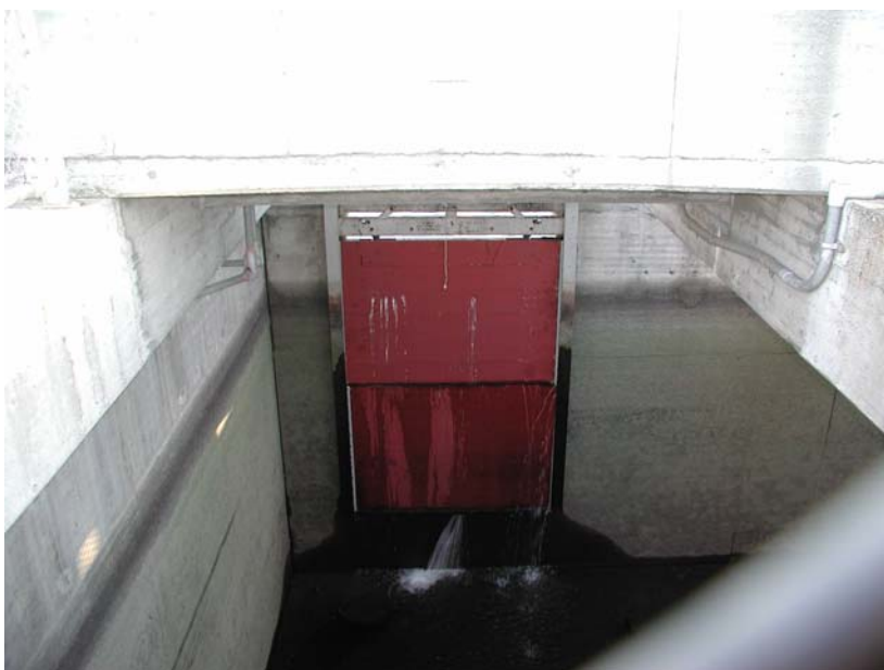
Figure 4c. Red gate is the adult fish exit from the fish ladder. This photograph was taken during the winter maintenance period when the ladder was dewatered in 2003.
