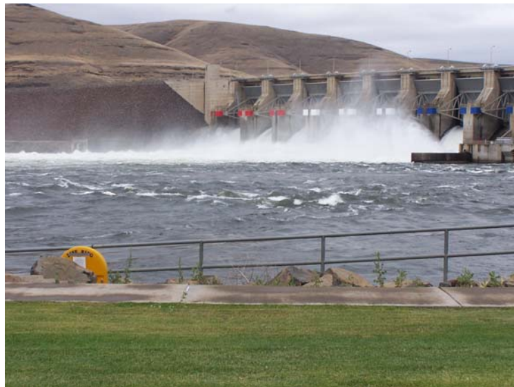
Figure 6c. June 28 spill at Little Goose Dam that slowed or stopped passage of adult salmon for nearly 10 day until daytime spill level was reduced to about 30% of flow.
