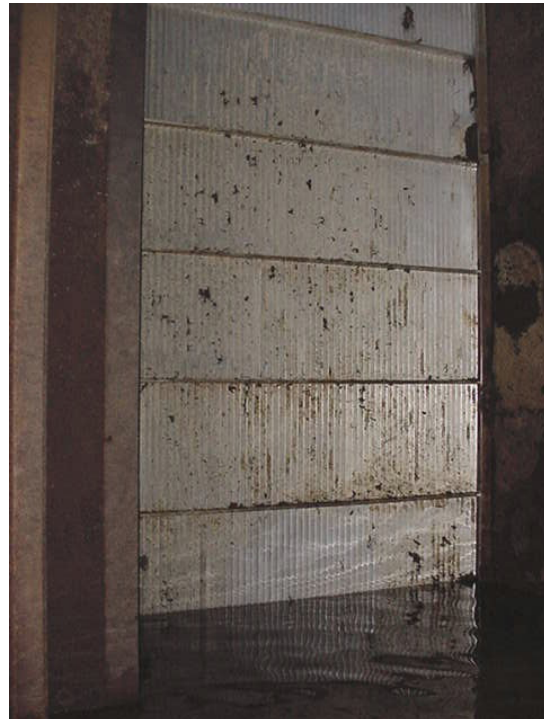
Figure 10d. AWS screen cleaning took about 6 hours (including dewatering the ladder and removing the adult fish from the upper pool). The fish ladder was immediately watered up and fish passage continued.
